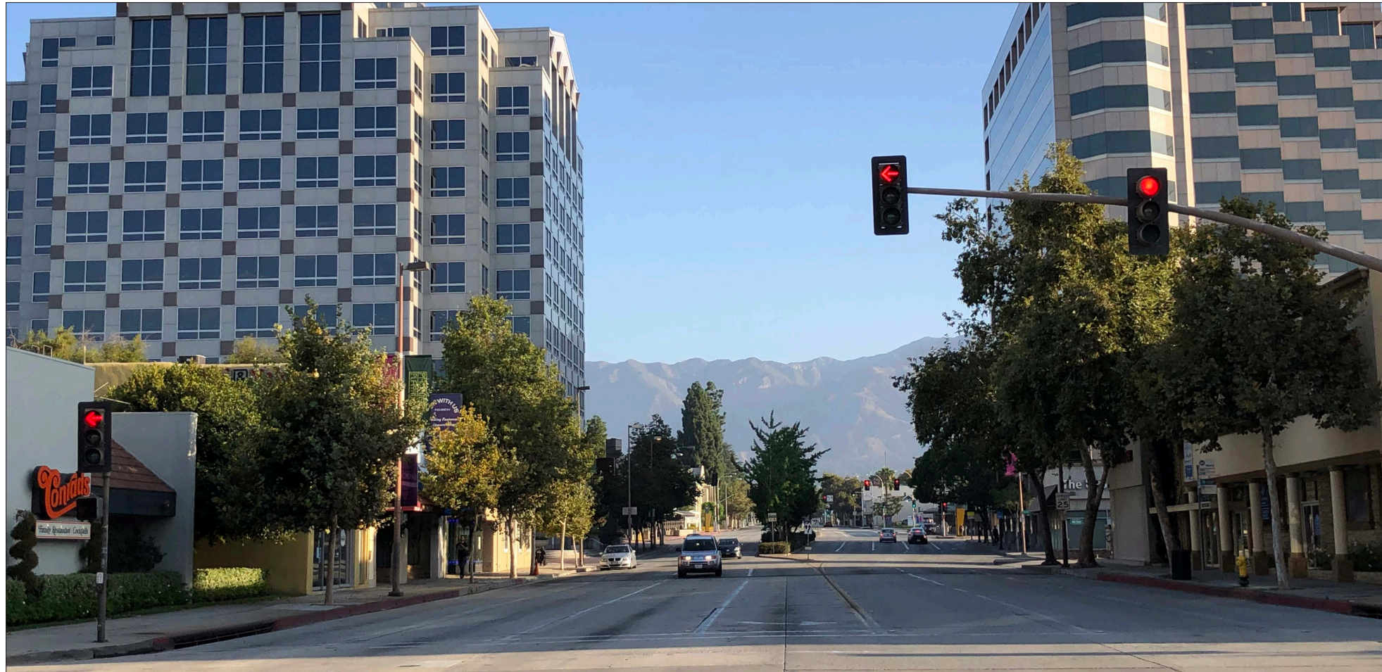
Lake Avenue existing conditions looking North
