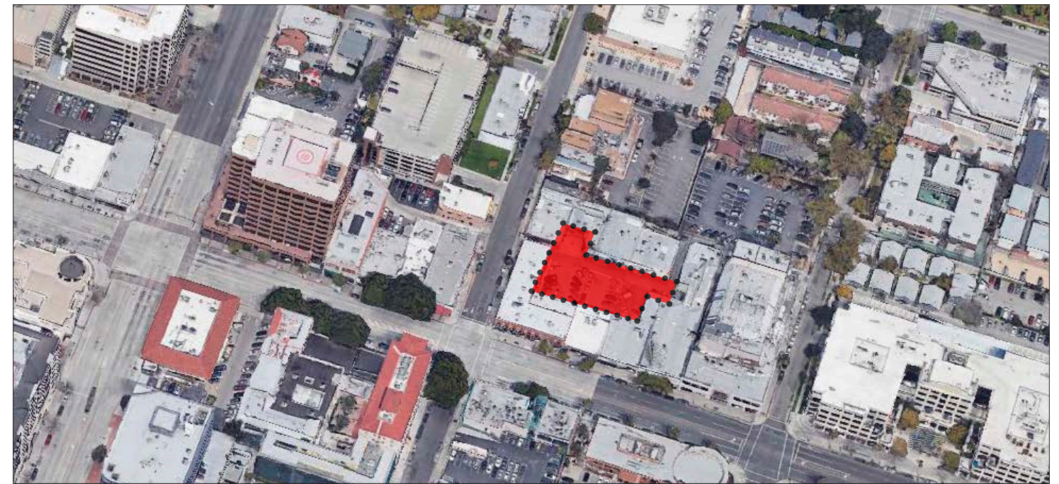
Parking lot with potential to become a plaza similar to One Colorado in Old Pasadena
