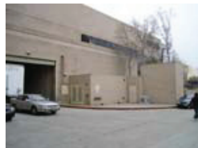
Loading dock for Paseo Colorado on Green Street
