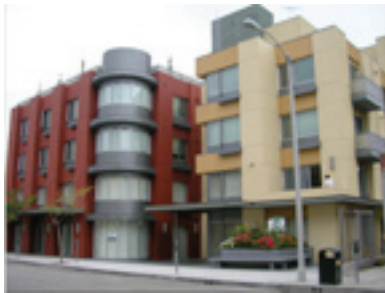
Messina Mixed-use Project in Old Pasadena provides new housing and commercial space
