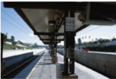
Lake Ave Station at freeway
