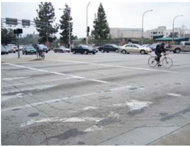
Poorly marked pedestrian crossing at Lake Avenue and Corson Street
