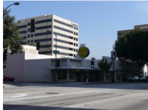
The 1-story buildings on the site have become outdated and do not take advantage of this important location.
